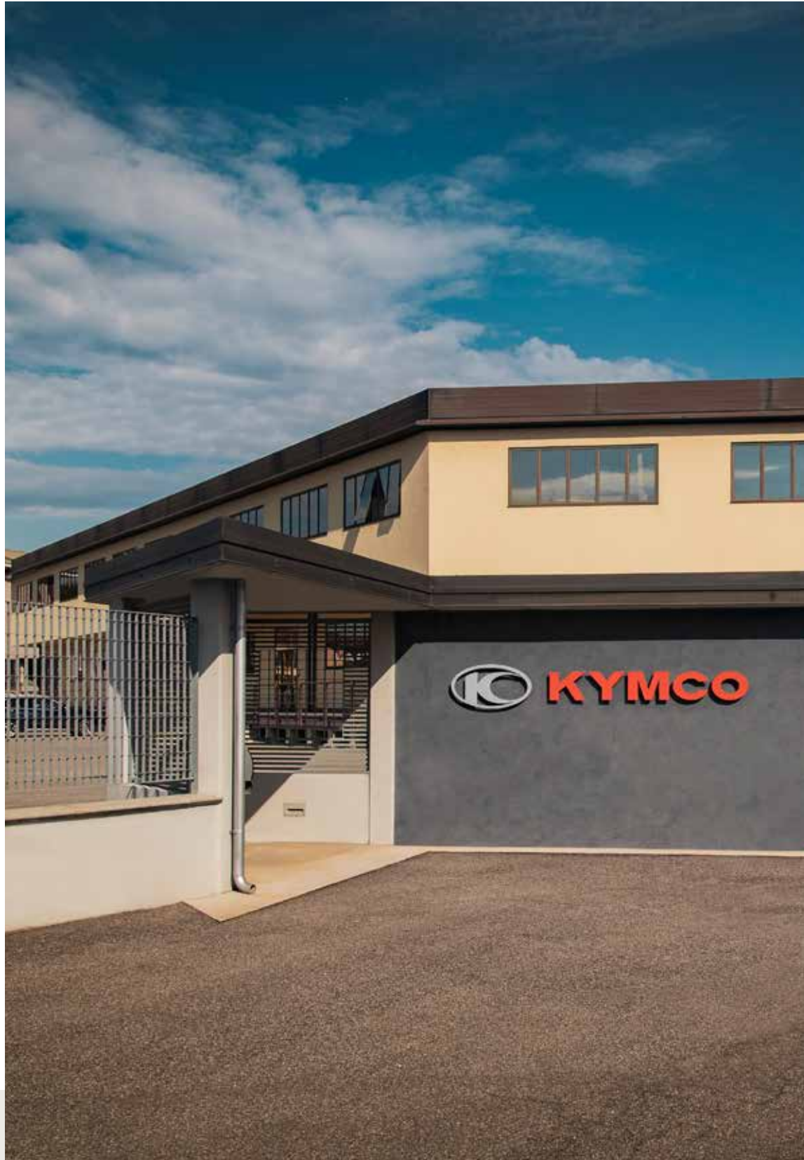
1. OFFICES & SPARE PARTS WAREHOUSE The settlement's estate area is about 6.100 m2; the factory's area is about 1.900 m2 . Outside area (4.200 m2) is used as parking, internal traffic and space for manoeuvre.
