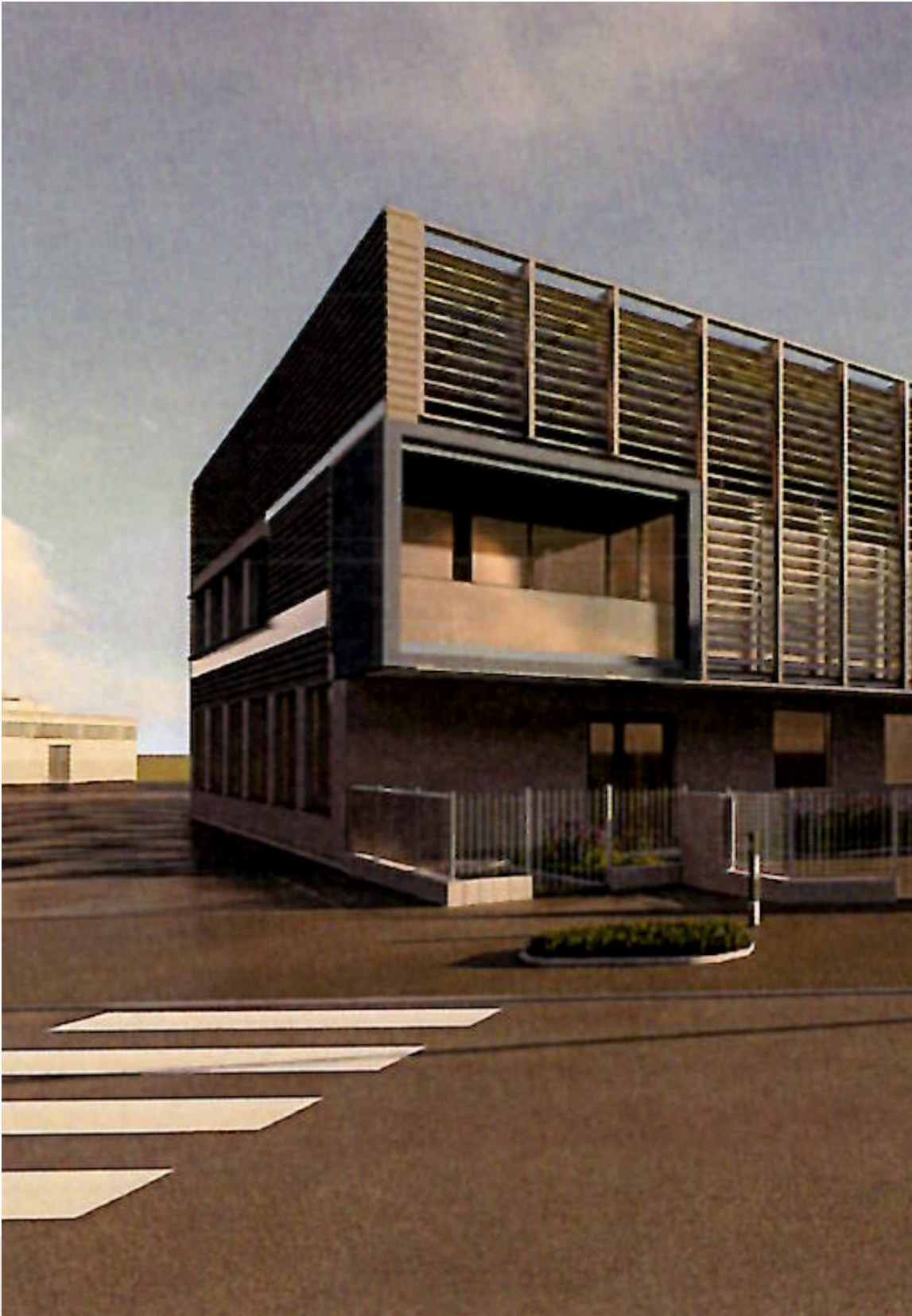
3. R&D DEPARTMENT The settlement's estate area is, according to land registry, 3.100 m2; the building occupied an area of about 2.800 m2.
